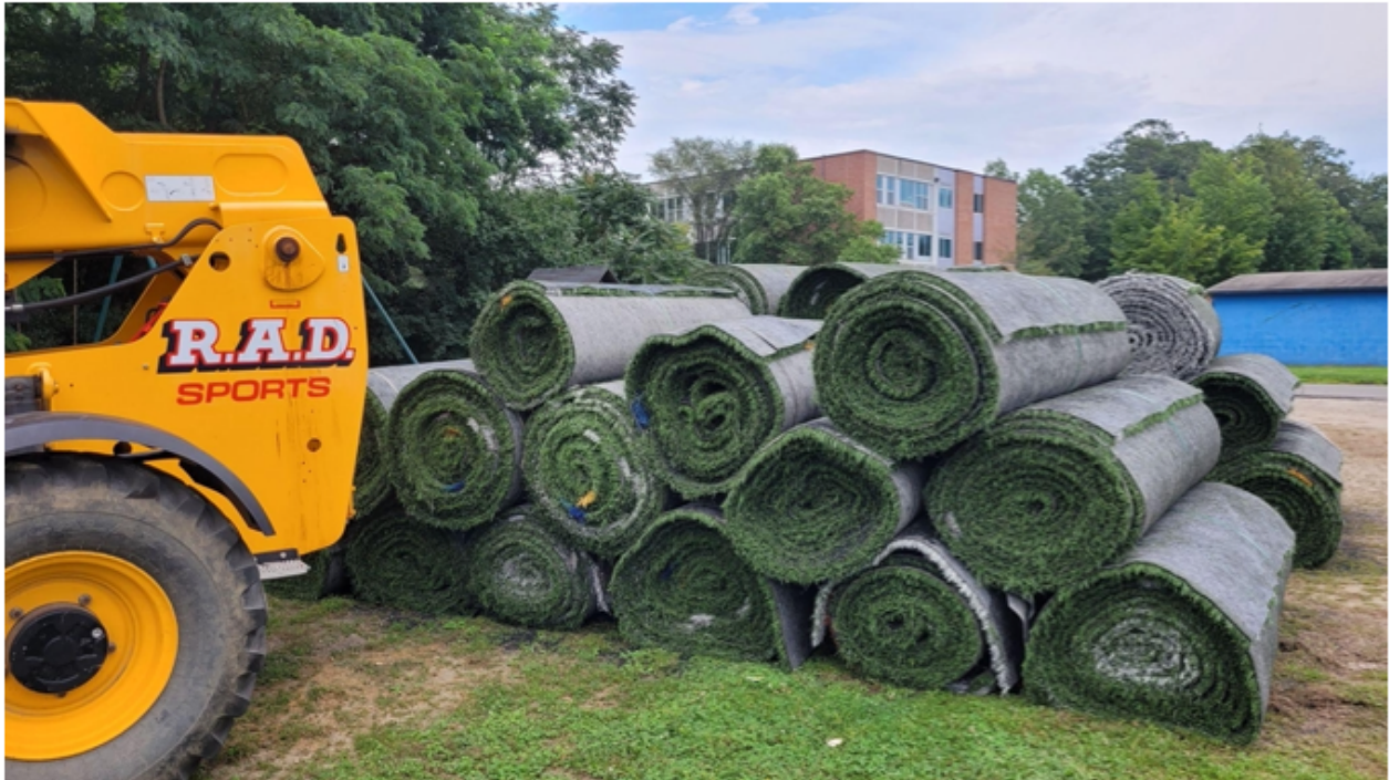
Old turf and fill material lying on unprotected ground
