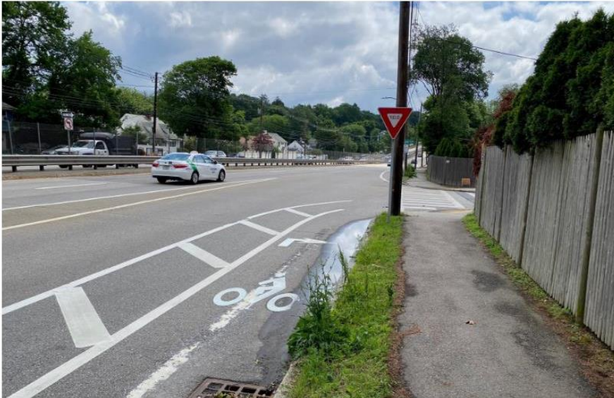
Boylston looking east at Sheldon Road
