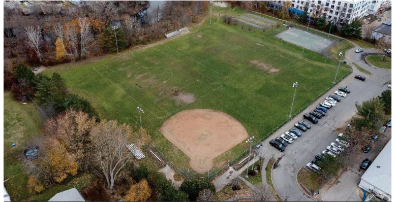
FORTE PARK MULTIPURPOSE SYNTHETIC TURF RETROFIT
