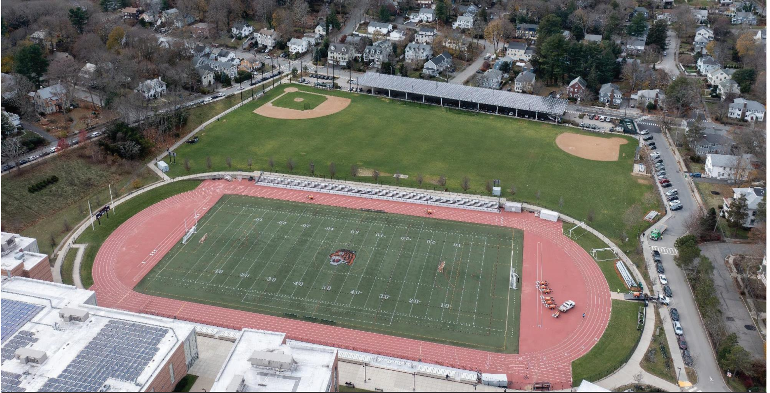
NNHS STADIUM SPORTS LIGHTING
