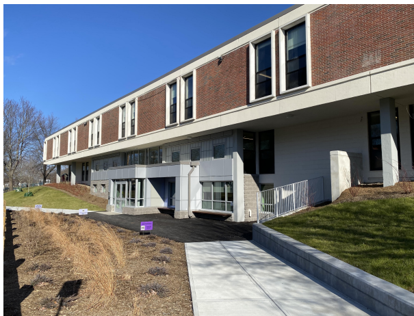
New Main Entrance on Albemarle Road
