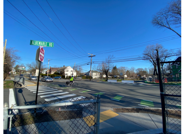
Pictured: Crafts Street at Albemarle Rd East northbound road closure.
