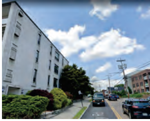
1. View down Langley Rd looking north
