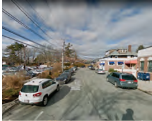
2. Wyman St at Waban T parking lot
