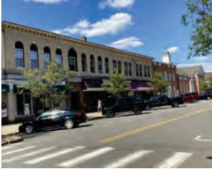
2. View down Auburn Street
