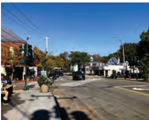
2. View down Walnut St looking north
