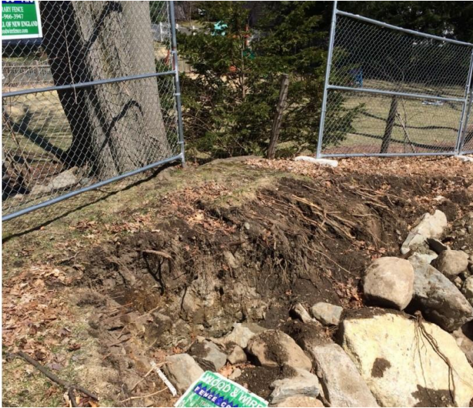
224 Melrose, Auburndale - tree roots damaged by 10 Elberta Terr construction
