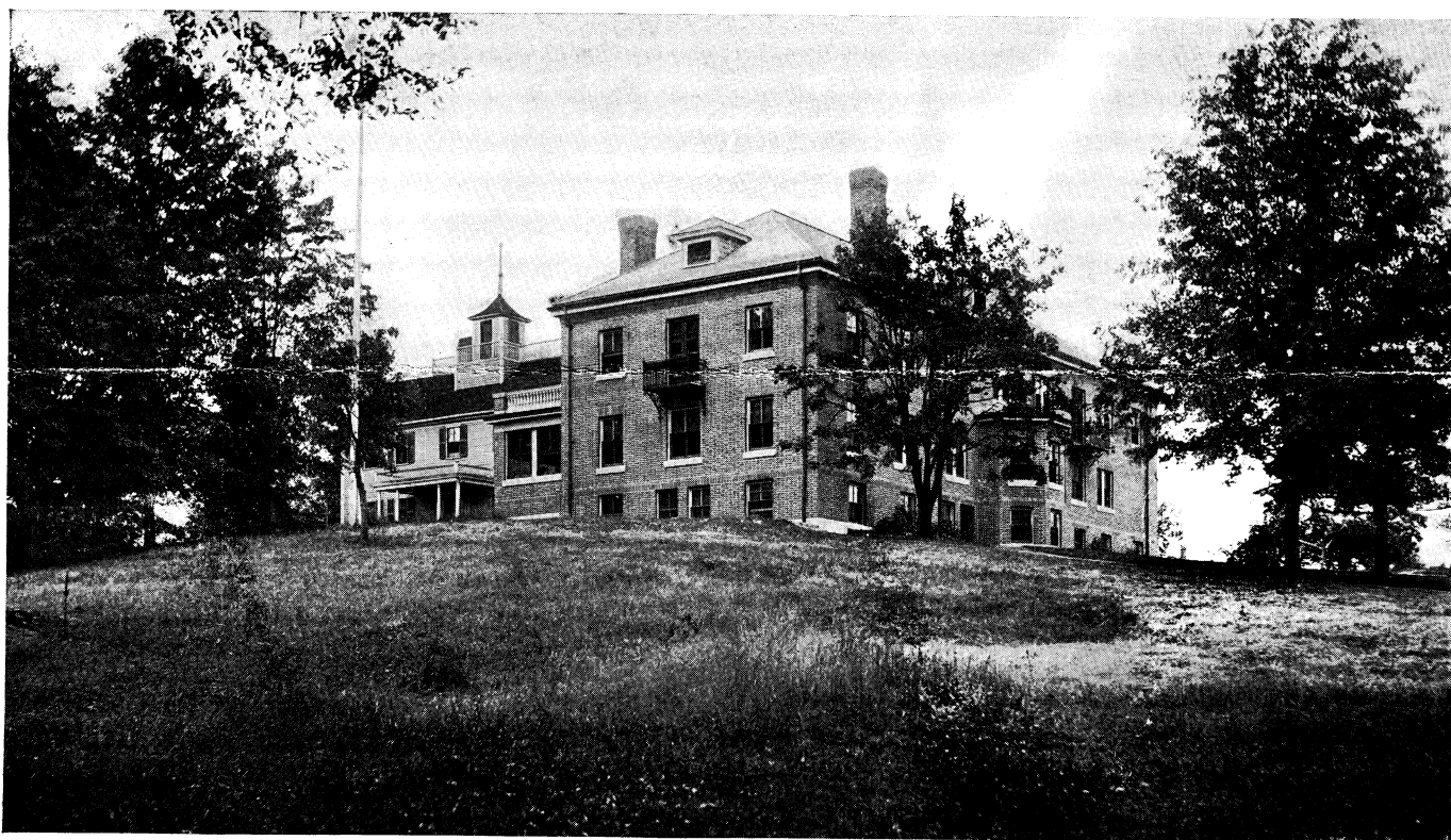
OLD HOME AND NEW EAST WING—SOUTH EAST VIEW
