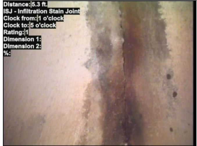
Photo: CATCH BASIN-T-STATION-5_6_2020 12_59 PM-ISJ-5.3 ft.-5_6_2020 1_01 PM.JPG
