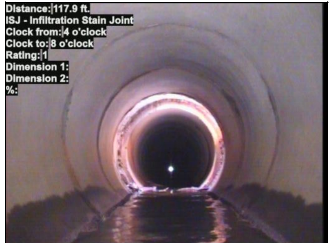
Photo: 337 GROVE ST MANHOLE-T STATION-5_6_2020 12_47 PM-ISJ-117.9 ft.-5_6_2020 12_54 PM.JPG
