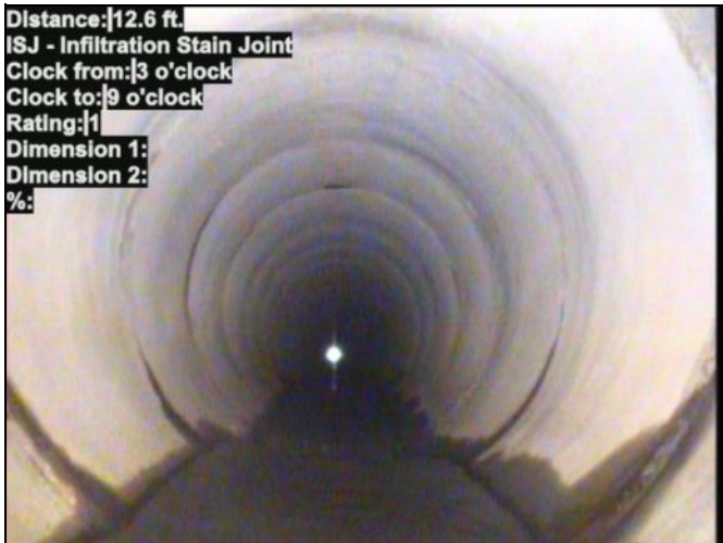
Photo: CATCH BASIN-T-STATION-5_6_2020 12_59 PM-ISJ-12.6 ft.-5_6_2020 1_02 PM.JPG
