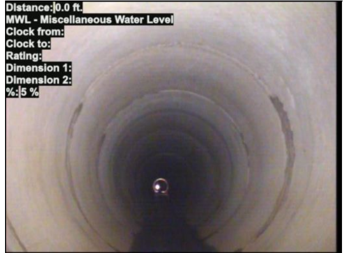
Photo: 337 GROVE ST MANHOLE-T STATION-5_6_2020 12_47 PM-MWL-0.0 ft.-5_6_2020 12_47 PM.JPG
