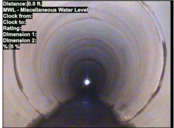
Photo: T-STATION-MH3-T-STATION-MH4-5_6_2020 1_14 PM-MWL-0.0 ft.-5_6_2020 1_14 PM.JPG
