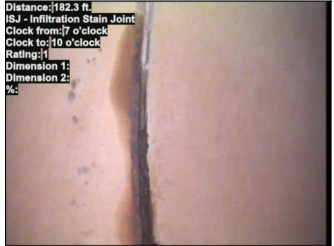
Photo: T-STATION-MH2-T-STATION-MH3-5_6_2020 1_08 PM-ISJ-182.3 ft.-5_6_2020 1_12 PM.JPG
