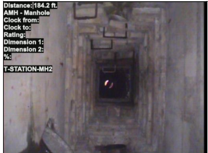
Photo: CATCH BASIN-T-STATION-MH2-5_6_2020 12_59 PM-AMH-184.2 ft.-5_6_2020 1_05 PM.JPG
