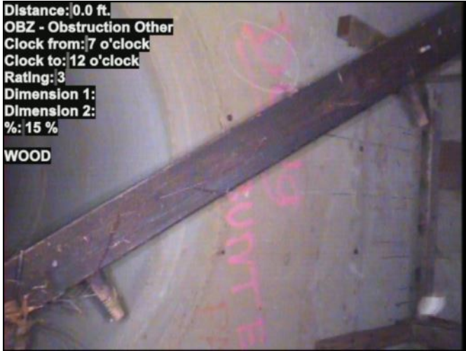
Photo: T-STATION-MH4-T-STATION-MH5-5_6_2020 1_19 PM-OBZ-0.0 ft.-5_6_2020 1_21 PM.JPG
