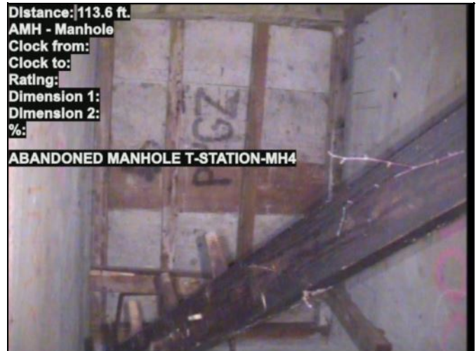
Photo: T-STATION-MH3-T-STATION-MH4-5_6_2020 1_14 PM-AMH-113.6 ft.-5_6_2020 1_18 PM.JPG
