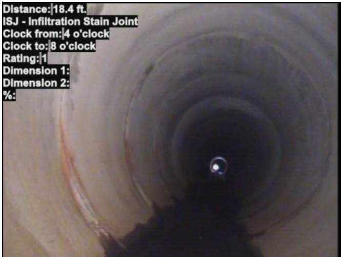
Photo: 337 GROVE ST MANHOLE-T STATION-5_6_2020 12_47 PM-ISJ-18.4 ft.-5_6_2020 12_52 PM.JPG
