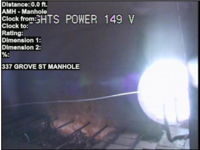
Photo: 337 GROVE ST MANHOLE-T STATION-5_6_2020 12_47 PM-AMH-0.0 ft.-5_6_2020 12_47 PM.JPG
