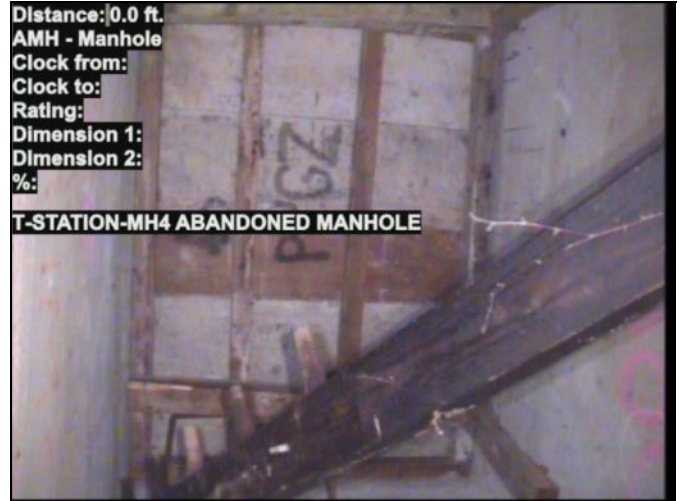
Photo: T-STATION-MH4-T-STATION-MH5-5_6_2020 1_19 PM-AMH-0.0 ft.-5_6_2020 1_20 PM.JPG
