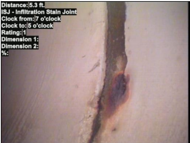
Photo: T-STATION-MH3-T-STATION-MH4-5_6_2020 1_14 PM-ISJ-5.3 ft.-5_6_2020 1_15 PM.JPG
